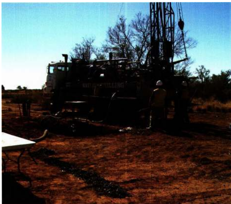
Drilling at Maree
